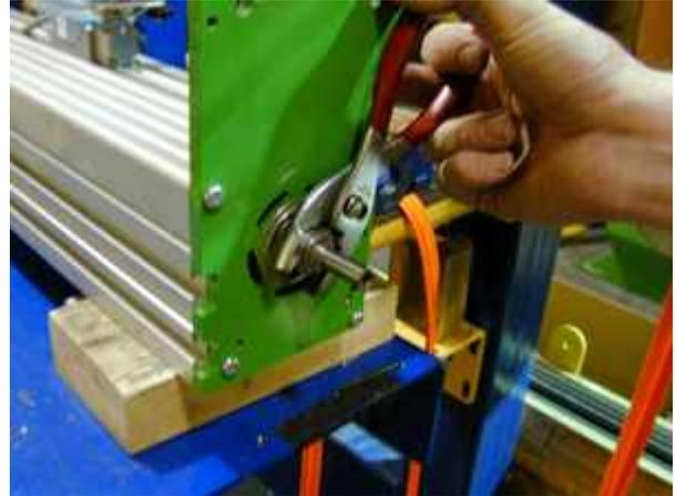
Tightly grip the lock nut at the motor end of the drive screw with a pair of pliers, and rotate it until it can be removed. (It's threaded onto the screw.) ▶
